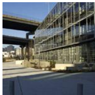
Along the southern side of the RiverEast Center , a normal asphalt street was replaced with a semi-permeable public plaza that aggregates rainwater from collection systems around the site. Photo: David Owen / Artifice Images
