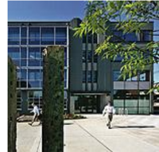
Sections of concrete wall, removed to add windows and improve daylighting throughout the RiverEast Center , were reused in a site installation designed by artist Linda Wysong. Photo: Gary Wilson Photo/Graphic
