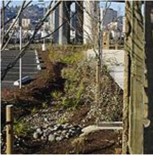
Swales collect rainwater from the parking lot adjacent to the RiverEast Center . Photo: David Owen / Artifice Images
