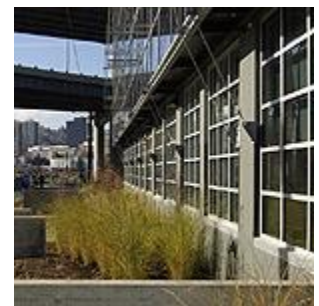
Salvaged sections of concrete wall were reused throughout the RiverEast Center 's sitewide rainwater collection system. Photo: David Owen / Artifice Images
