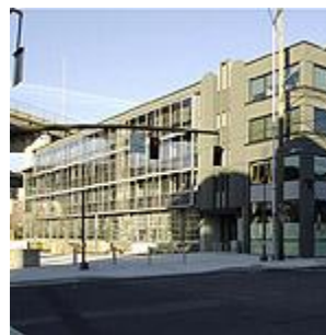
As much as 30 percent of the existing wall concrete was replaced with windows during the renovation of RiverEast Center . Photo: David Owen / Artifice Images
